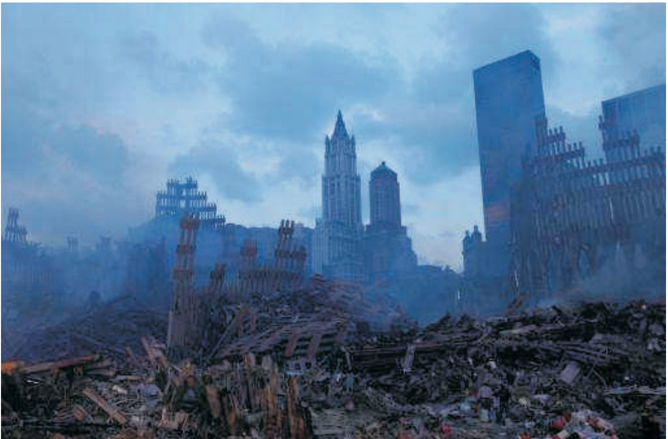
Figure 12-1.—"Ground Zero" at the site of the World Trade Center terrorist attack, September 11, 2001.
